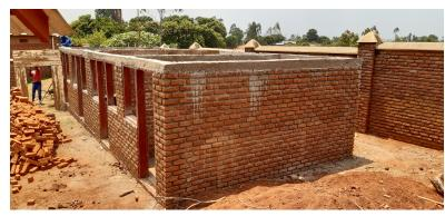
Once these rooms were up to the ring beam, we felt to do the other 2 rooms before doing the ring beam. We finished the other 2 rooms and the ring beam last week. We have enough
